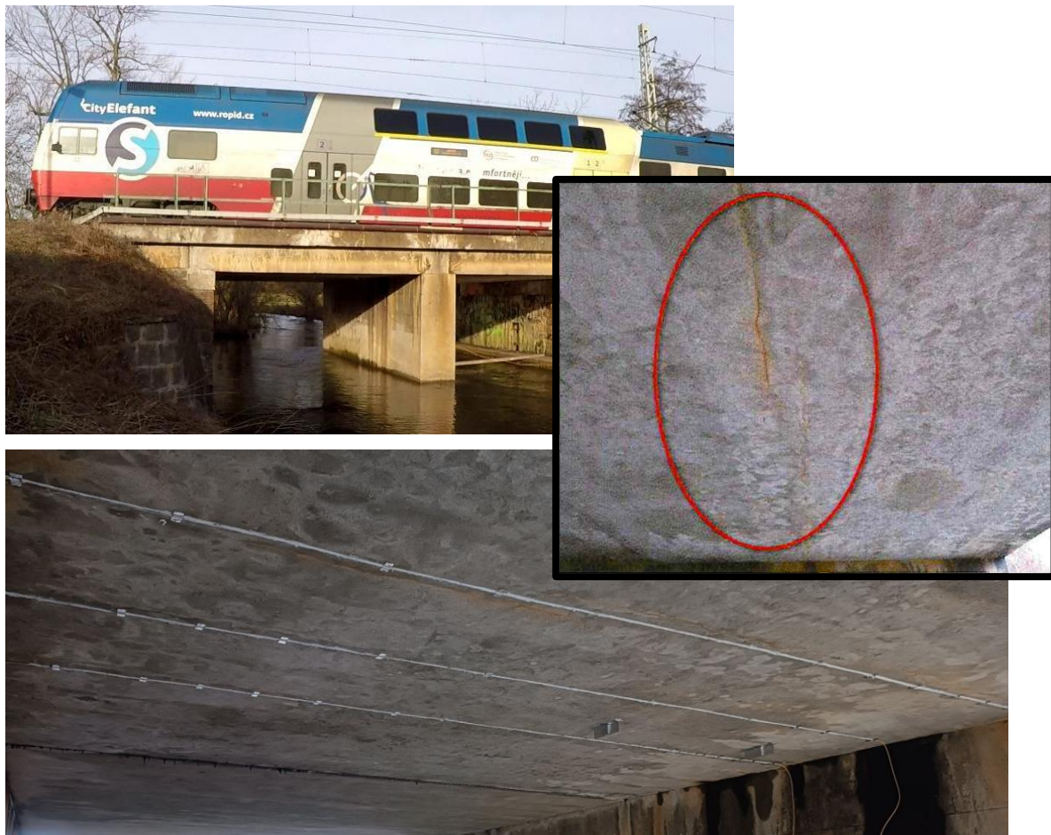
Fig. 11: Railway bridge in Kostomlaty, Czech Republic, showing the observed damages and the installed FBG monitoring system.
